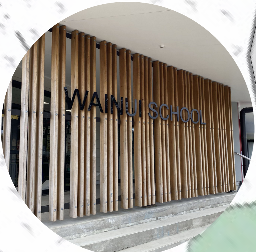
Existing screen on hall
